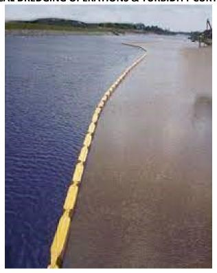
Image by One Clarion. Example of a turbidity curtain containing suspended sediment, as shown by the darker shade of the water inside the curtain as compared to outside the curtain.
