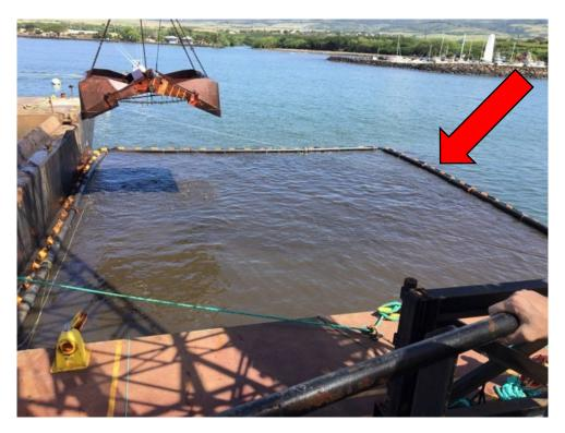
Image by USACE. A dredge bucket is being lowered into work area that is surrounded by a turbidity curtain. A turbidity curtain contains any sediment (mud and sand) that may be suspended in the water, as shown by the darker shade of the water inside the curtain as compared to outside the curtain.
