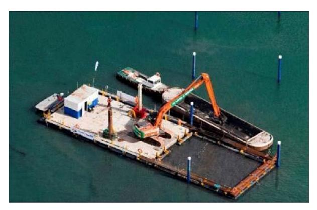
Image by Semantic Scholar. Typical dredging operation is comprised of an excavator mounted on a barge that removes dredged material within a turbidity curtain perimeter and transfers it to a nearby scow barge for transport. The scow barge is towed to a disposal site by a tug or support vessel.
