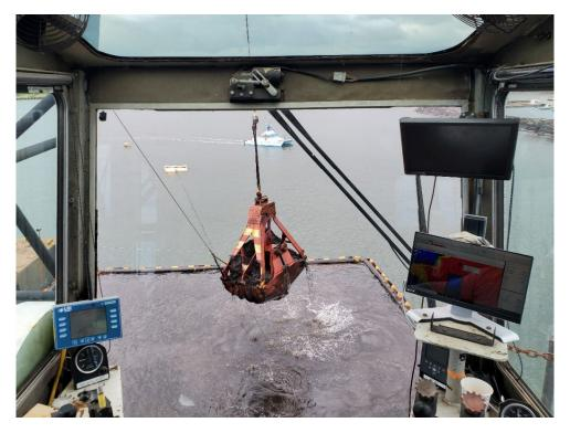
Image by USACE. Sediment is being removed by clamshell dredge bucket. A turbidity curtain contains any sediment (mud and sand) that may be suspended in the water, as shown by the darker shade of the water inside the curtain as compared to outside the curtain.
