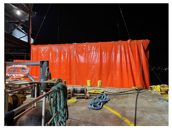
Image by USACE. The orange turbidity curtain being lifted out of the water.
